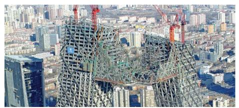
Figure 12. The Overhang before connection
