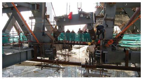
Figure 14. Installation of first connection element
