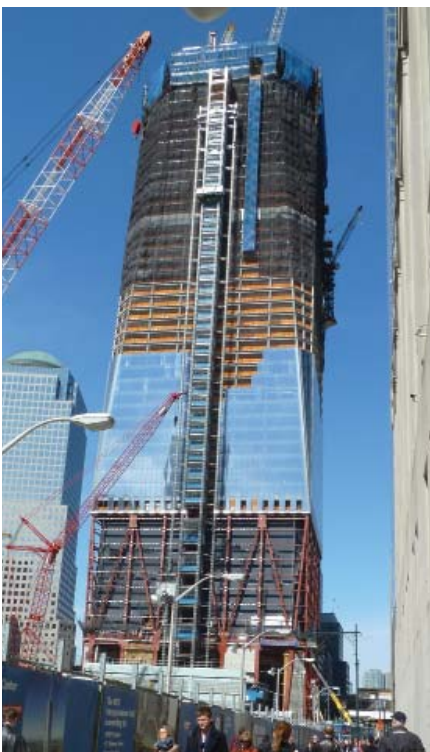
Figure 7. 1WTC under construction © Tansri Muliani
