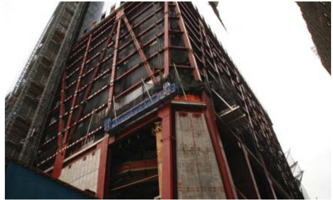
Figure 4. Structural steel moment frame at the tower perimeter © Jan Klerks
