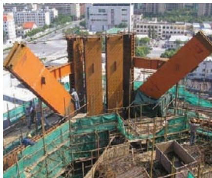
Figure 6. The diagonals of the mega-structure, formed from welded boxes of structural steel.
