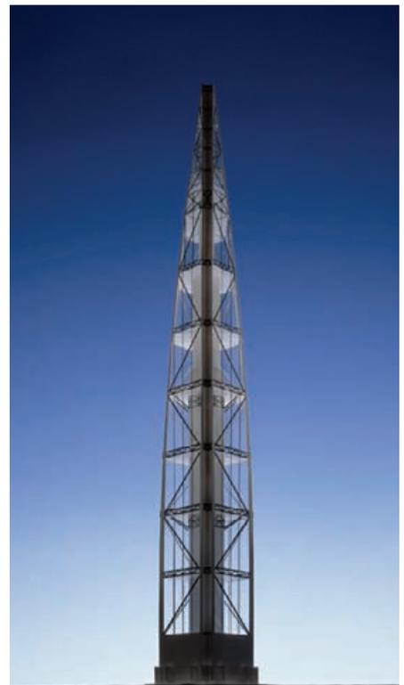
Figures 3 & 4. Model showing the building's mega-structure system of mega-columns, diagonals and belt trusses along with concrete core walls and outrigger trusses.
