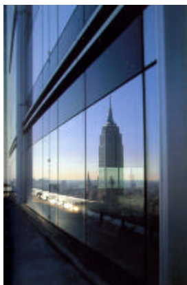
Fig.2. Photovoltaic Spandrel Panel, Four Times Square
